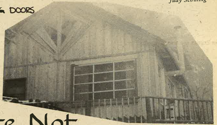
The hand-built house
