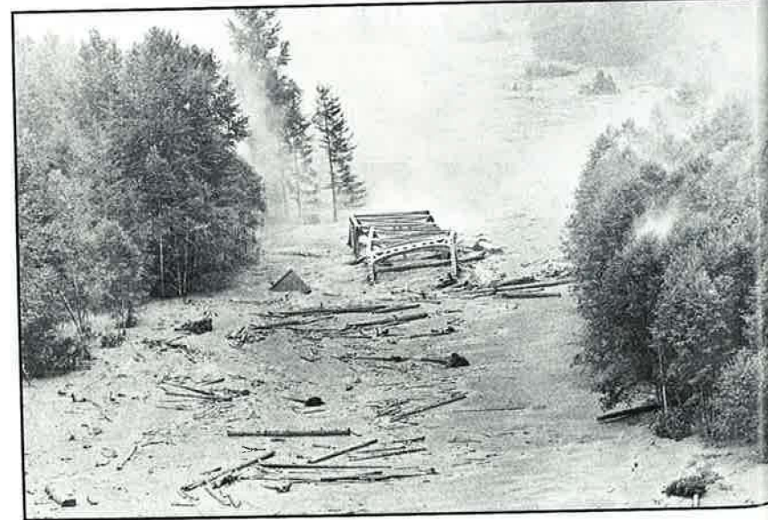
Battered by a 50 mph torrent of mud and fallen trees (top), this Spirit Lake Highway bridge across the North Fork of the Toutle River finally yields to the onslaught in this sequence of photos. The span bends (center) and is ripped from the banks and carried downstream (bottom), only to become part of the destructive flow (far right) it tried to resist.
