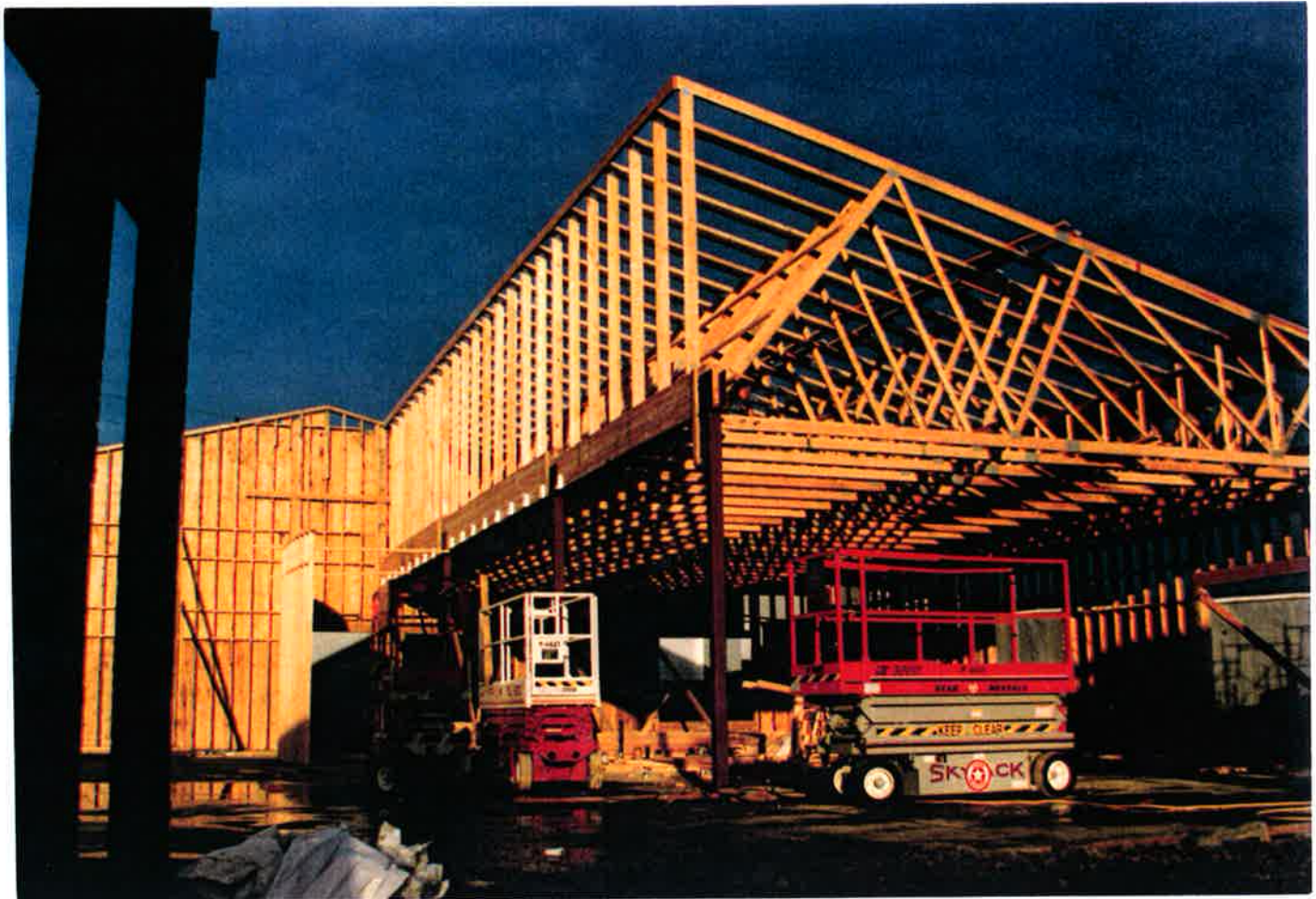
2. EARLY STAGE OF CONSTRUCTION.
