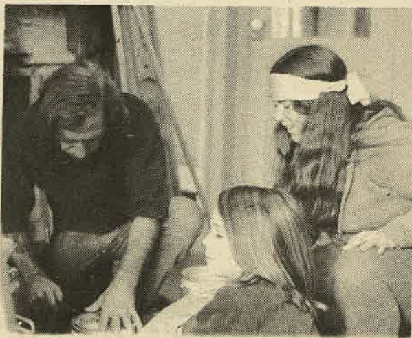
Bob Freeman (Head Start), Judy Schilling and Jason Schmidt at work on the Shelter Home
